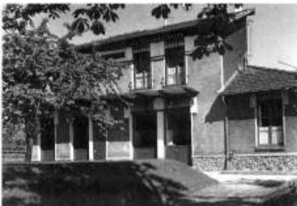
108. The annex of the Mureed's house, an old building renovated in the early thirties.
